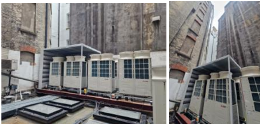
Figure 5: Photos of condensers with acoustic enclosure installed
