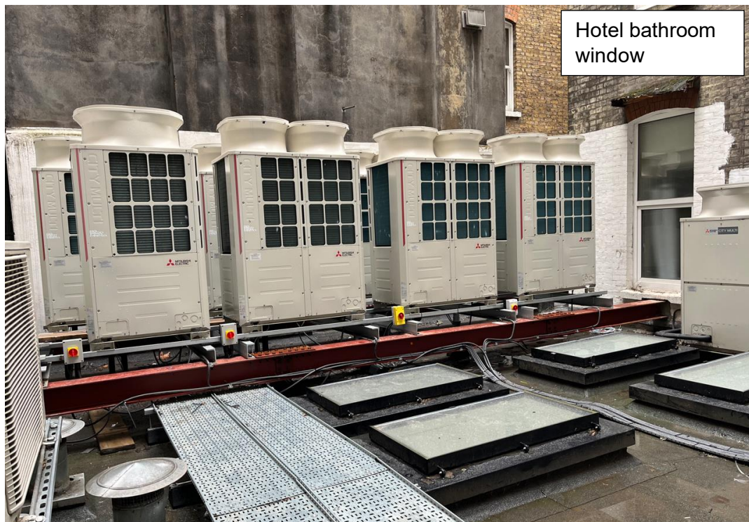
Figure 3: Views of condensers (as installed) prior to installation of acoustic enclosure
