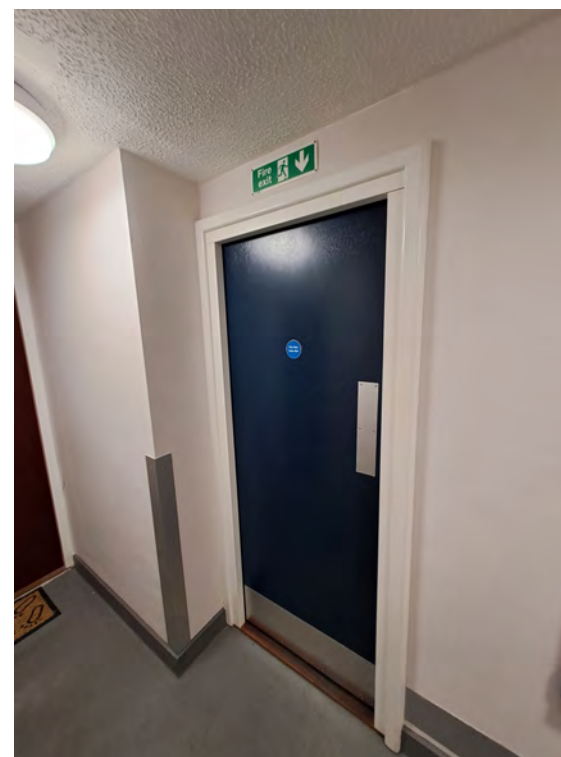
Fire door leading to stairwell at 6 Greville Street.
