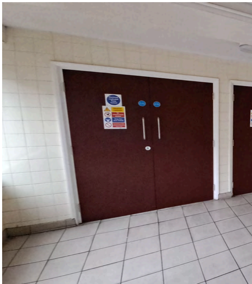
Service Riser Cupboard Fire Doors at Cartmel.
