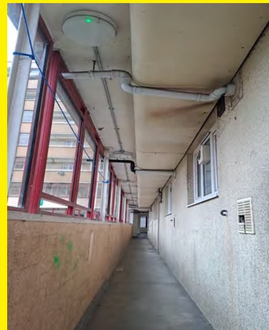
Emergency lighting on open access corridor at Cartmel.
