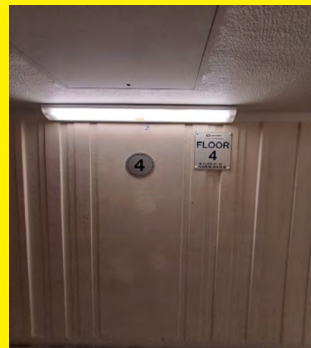
Emergency lighting on escape routes at Bray Tower.
