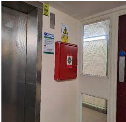
Secure Information Box at Bray Tower.
