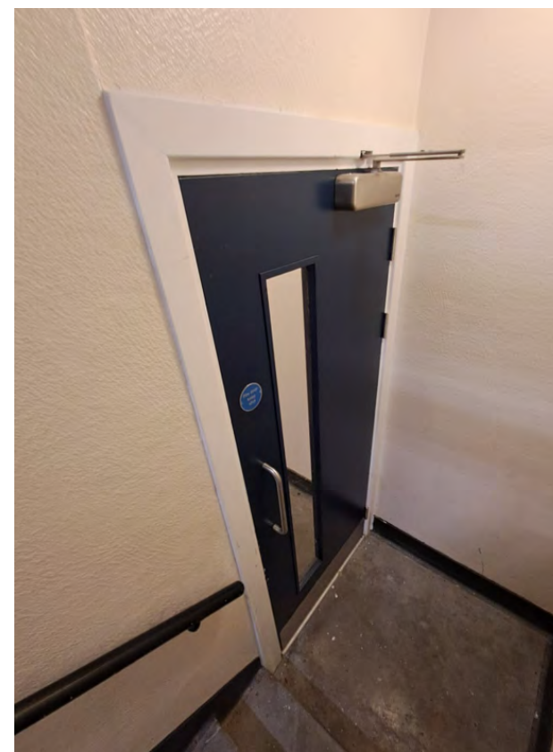
Communal Fire Door at 1-22 Rydal Water Hampstead.
