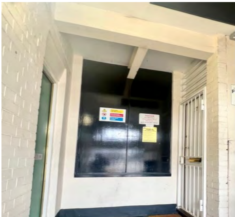
Electrical cupboard Fire door at Cavendish Mansions.
