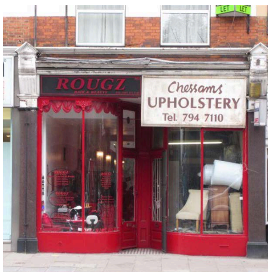
Photo 13: Victorian / Edwardian Shopfront at 483-485 Finchley Road
