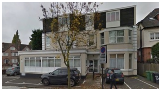
Photo 19: 1 Platt's Lane, Front Elevation
