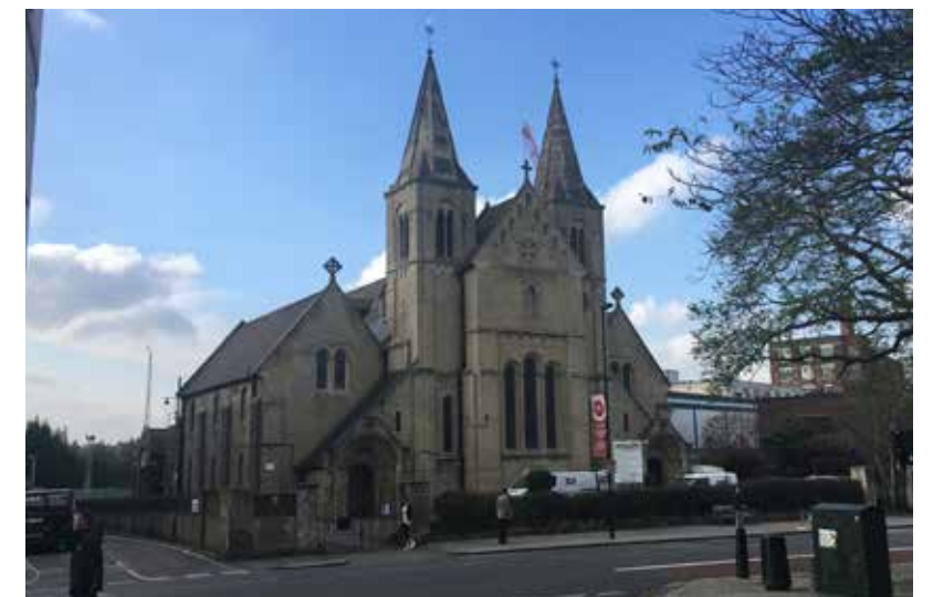
CHURCH OF ST JOHN, HIGHGATE ROAD, GRADE II LISTED
