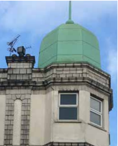
DOME, 189 KENTISH TOWN ROAD
