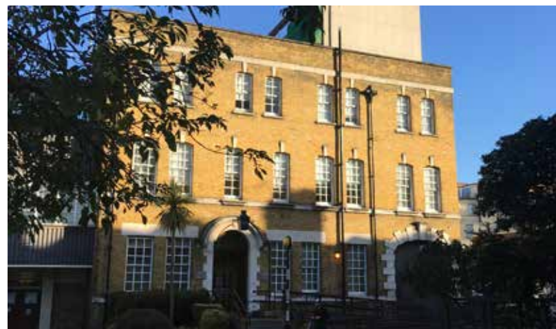
KENTISH TOWN POLICE STATION, GRADE II LISTED
