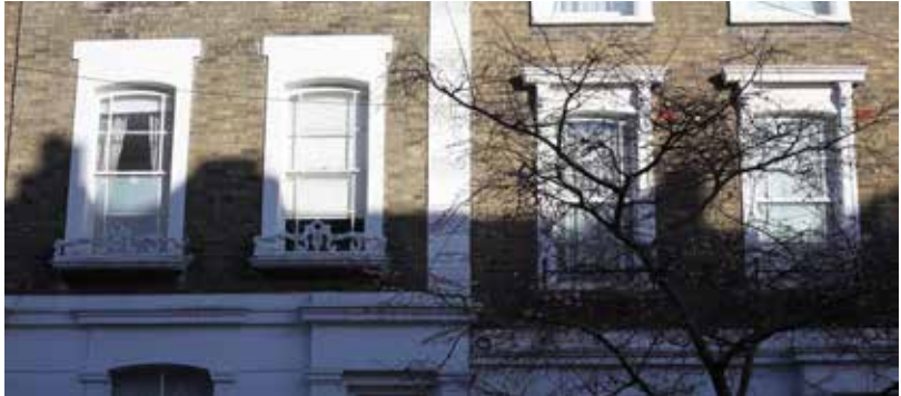
WILLES ROAD FACADES
