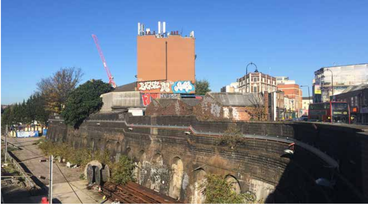
VIEW ACROSS RAILWAY CUTTING TOWARDS HIGHGATE ROAD
