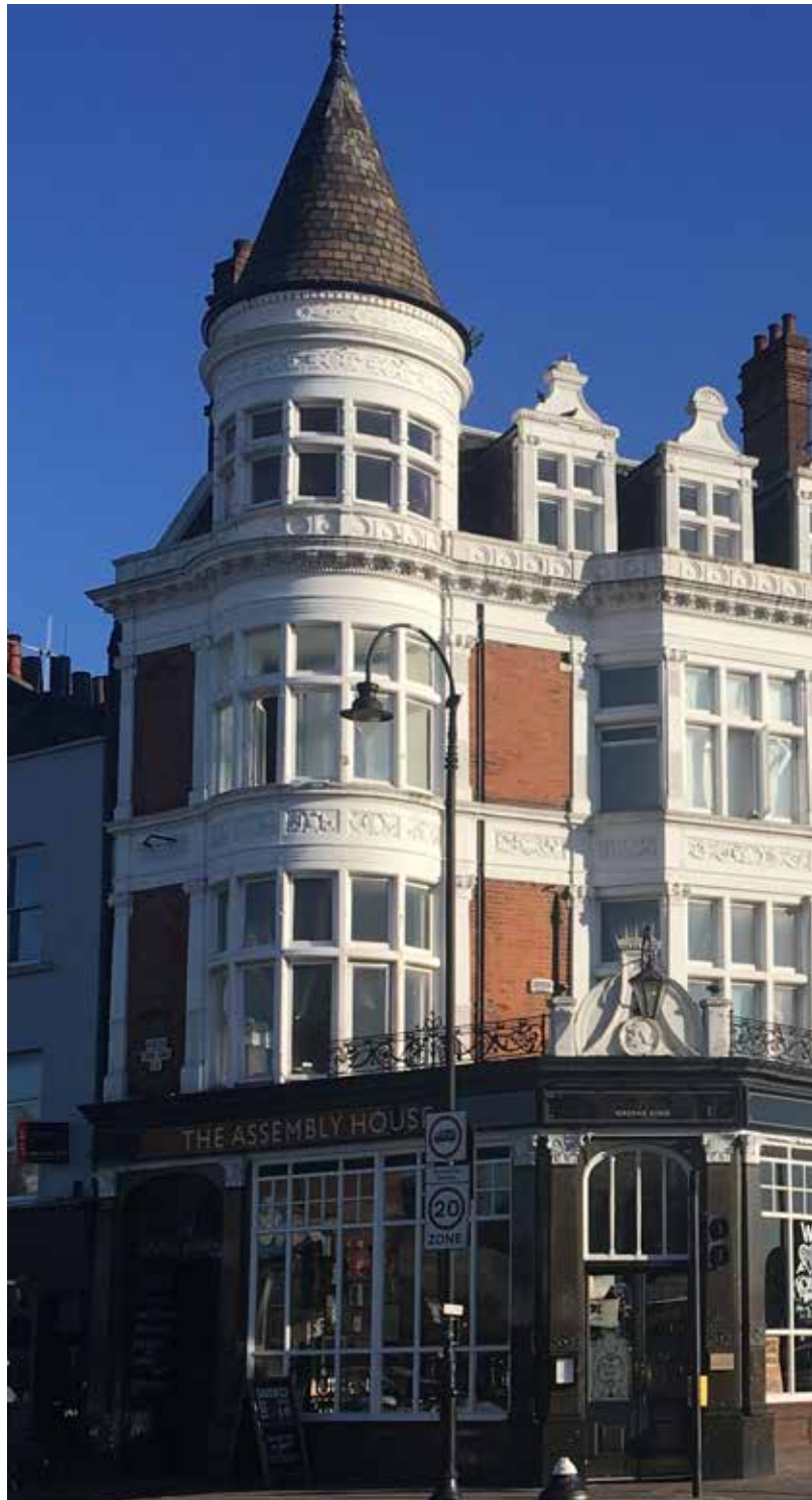
THE ASSEMBLY HOUSE, GRADE II LISTED
