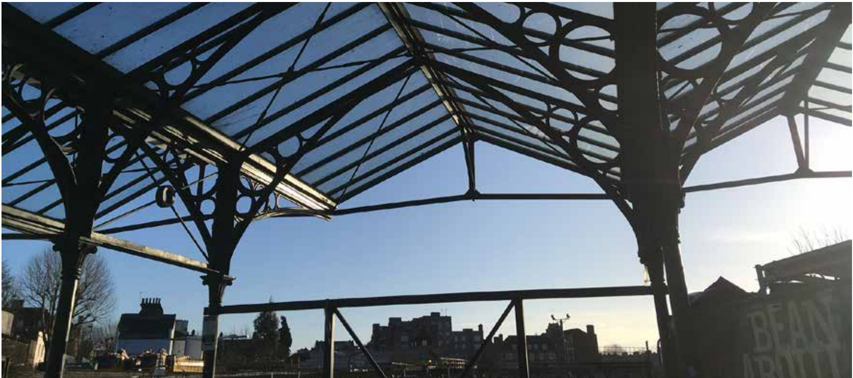
CANOPY AT KENTISH TOWN STATION
