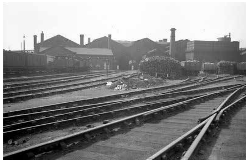
KENTISH TOWN LOCOMOTIVE SHEDS
