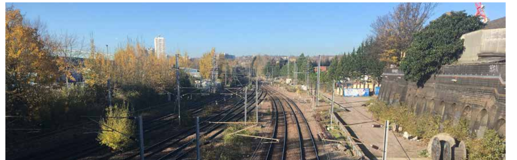
RAILWAY CUTTING RUNNING THROUGH KENTISH TOWN
