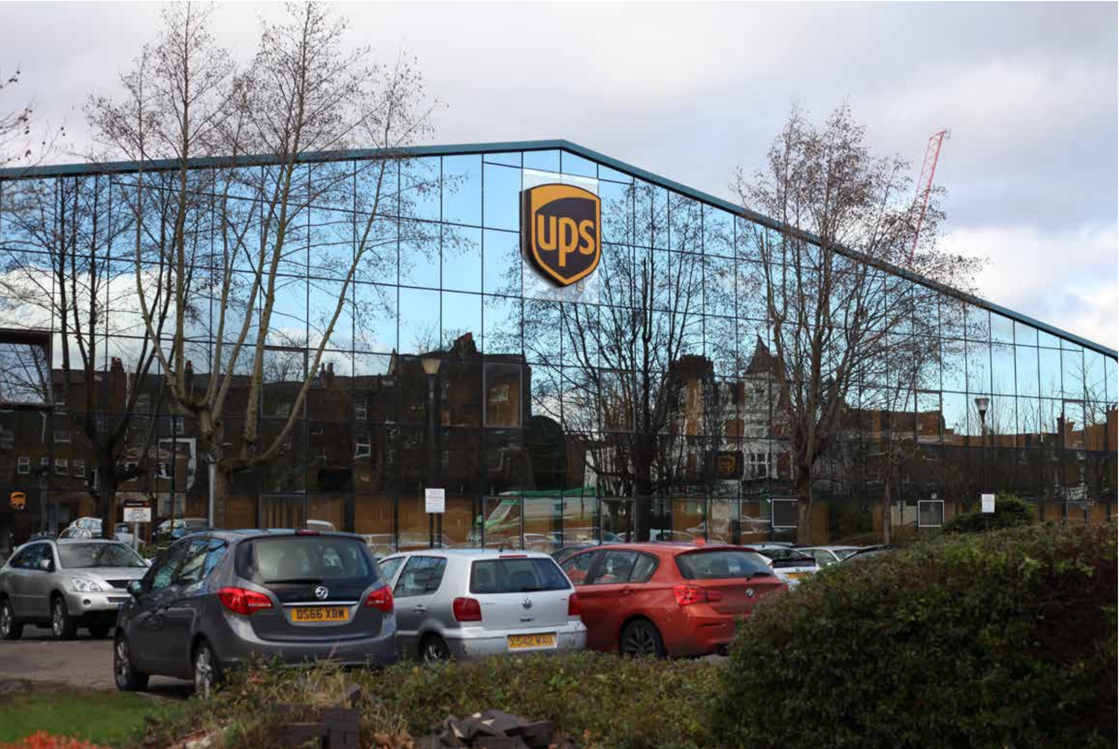
UPS, REGIS ROAD
