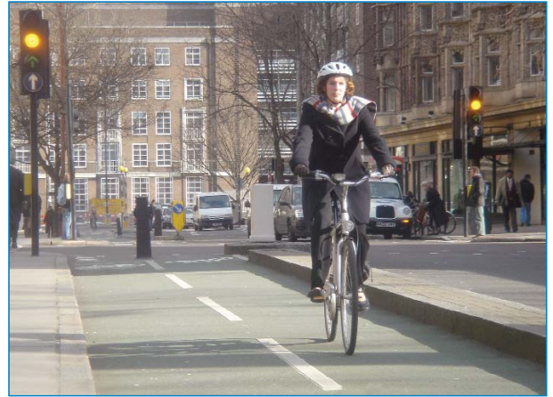
Segregated cycle lane in Torrington Place
