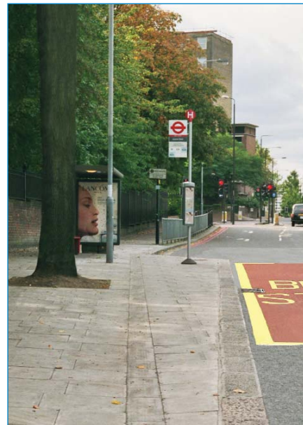
Obtuse bus boarder in Adelaide Road
