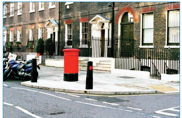
Footway build-out in John Street
