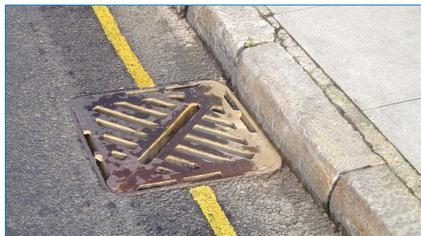
Carriageway gully cover – Double triangular D400
