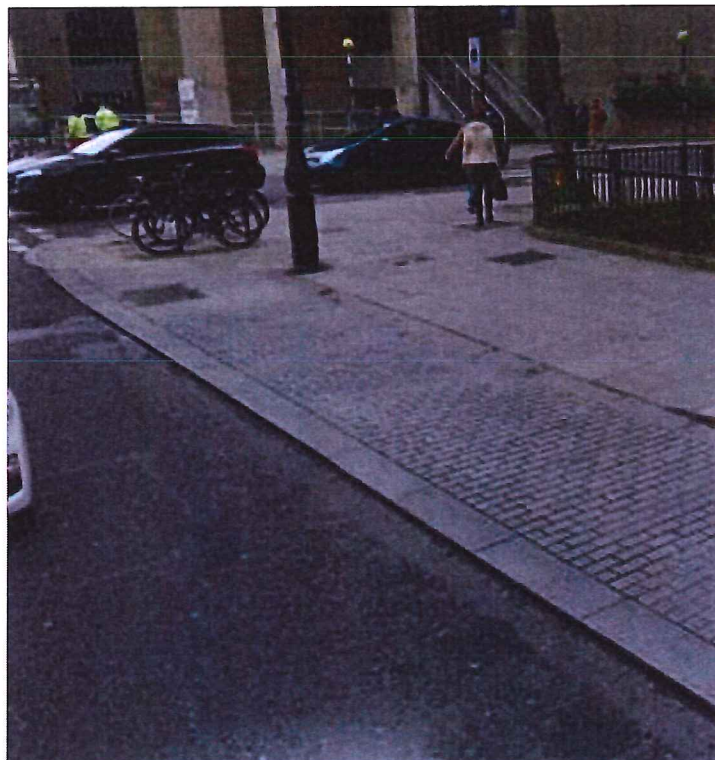
Example of half-kerbed inset taxi / loading bay on Russell Square
