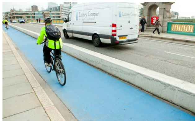
Kerbed separation, Southwark Bridge
