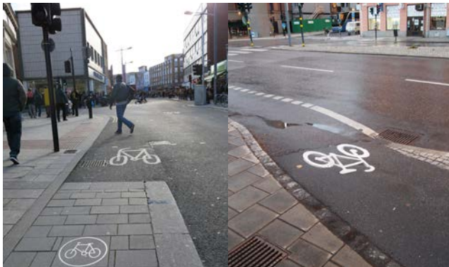
Transitions between on- and off-carriageway cycling: Rye Lane, Peckham (left) and Stockholm (right)
