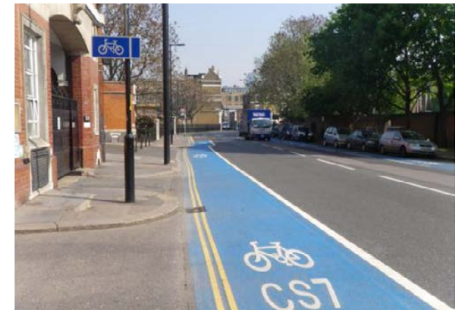
Mandatory cycle lanes, including an example of a sign to diagram 959.1 of TSRGD
