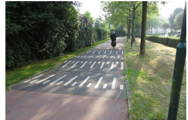
Double humps in Utrecht to prevent use of the route by powered two-wheelers
