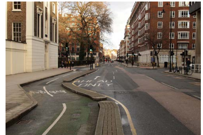
Track at Tavistock Street, Camden, forming a parallel carriageway and simplifying movement through a four-arm junction (but note the need for the left-turn ban).
