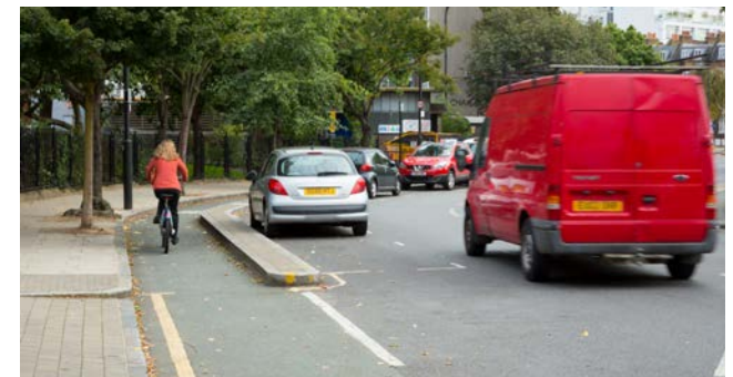
Cycle tracks at carriageway level that break to become lanes across accesses and side roads
