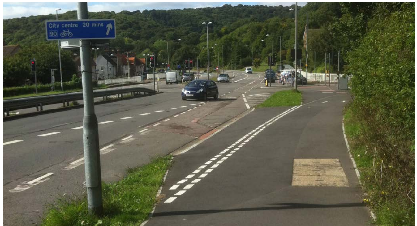
Long transition from on- to off-carriageway provision, with wide dropped kerb. Give way markings should not be used here
