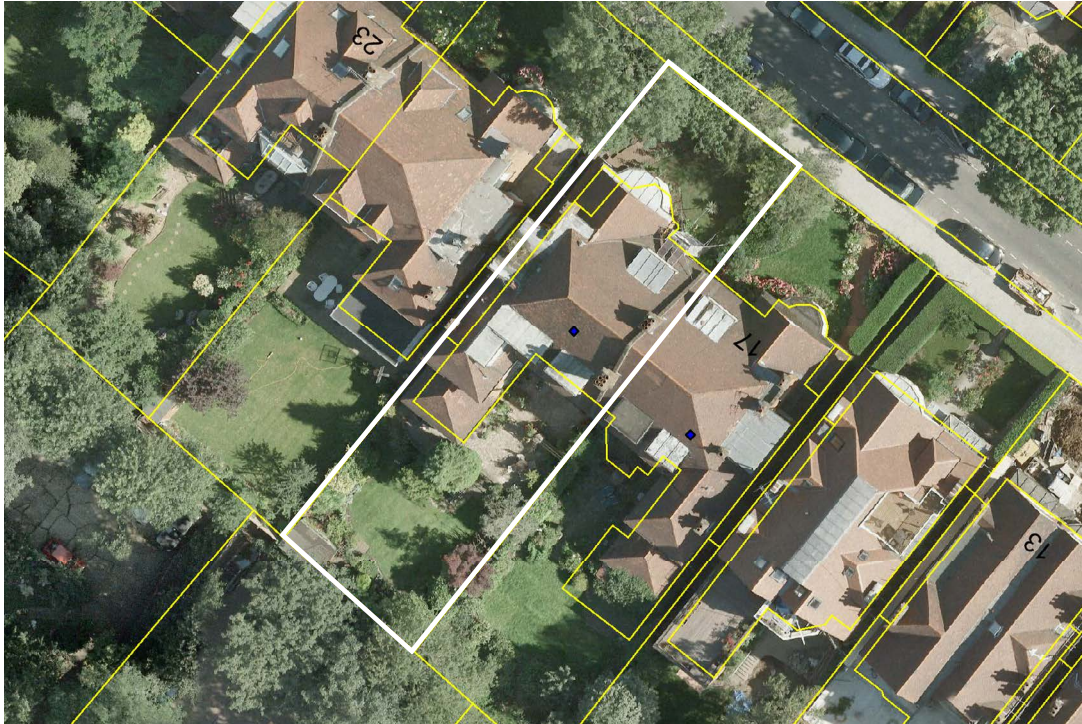
2007 Prior to construction of basement
