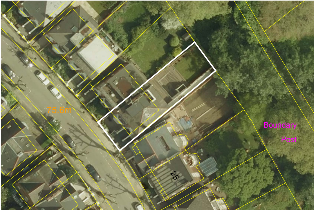
2014 Following construction of basement
