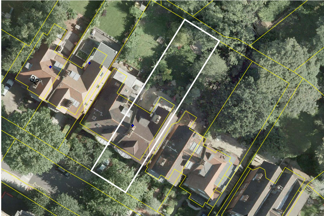
2007 Prior to construction of basement
