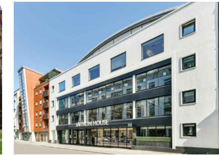
New development with EPC A rating - Saffron House in the Hatton Garden area (image credit: M&G)
