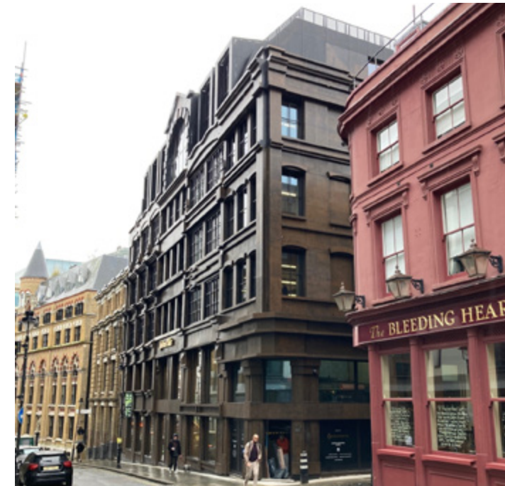
28 Greville Street, office refurbishment in Hatton Garden
