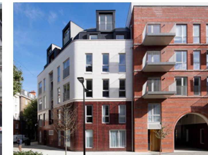
New development within Holborn's historic context - the Bourne Estate (photo credit: Benedict Luxmoore)
