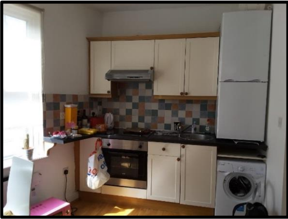
Inappropriate stacking of floor standing fridge freezer above washing machine
